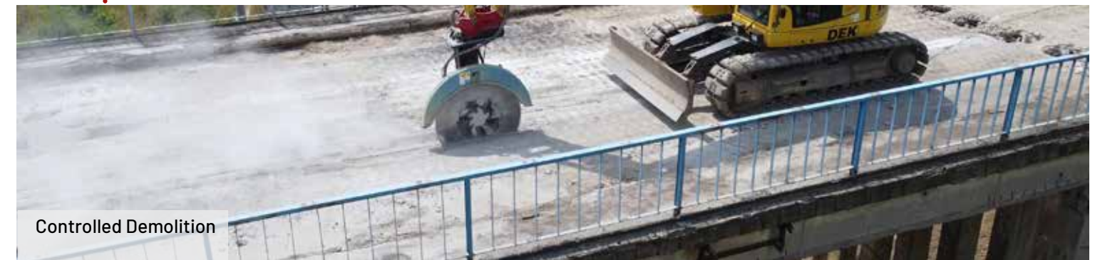
Foundation and plate cutting
