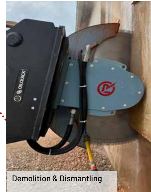
Foundation and plate cutting
